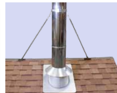
14. Support the chimney with an Extended Roof Bracket.
