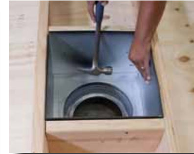
3. Nail the chimney support box to the framed opening from above. Use at least two 8 penny nails on each side.
