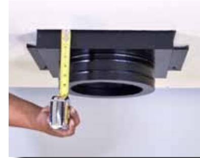
2. Slide the chimney support box into the framed opening from below, and level it. At least 2" of the box should extend below finished ceiling.
